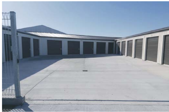
Hatrick Street East storage units
