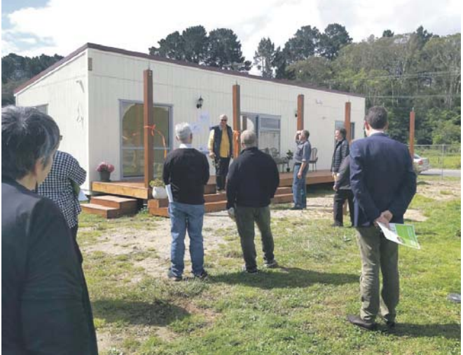
The front of the building awaiting completion of the veranda.
