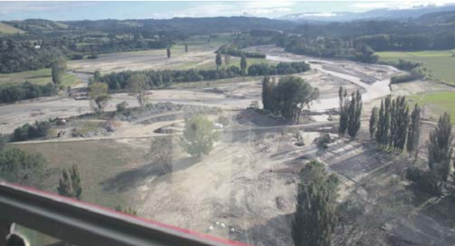
Aerial shot of damage on the Pohangina River following Cyclone Gabrielle.
