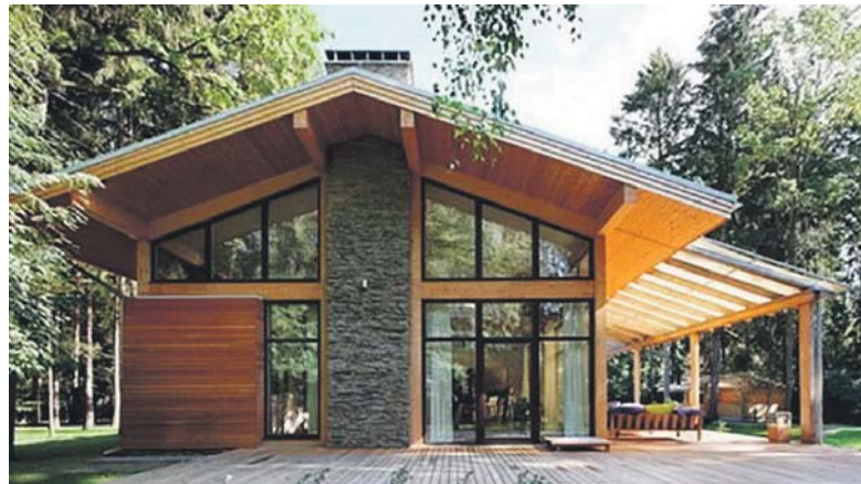
Wide eaves and pergolas can help keep your home cool in summer
