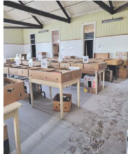
Fire extinguisher foam on damaged books
