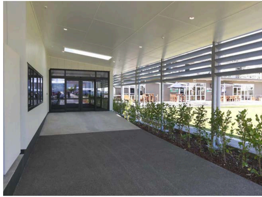
The new entrance leading into the St Johns Club from Wicksteed St.
