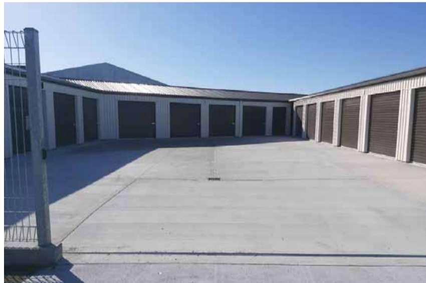
Hatrick Street East storage units
