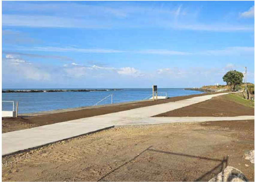
Tregenna Street works
