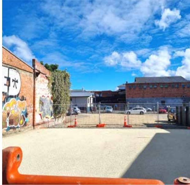
Progress being made with Corwen Park, Guyton St
