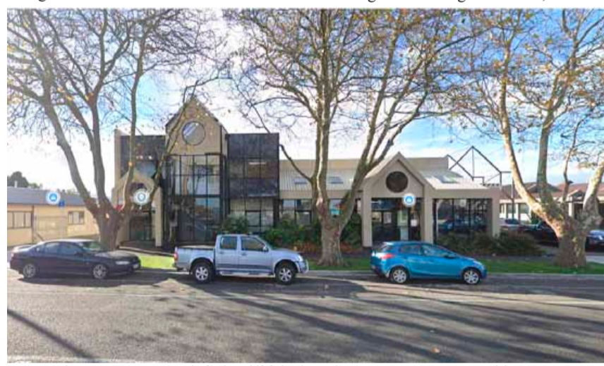
Alzheimers Whanganui, Suite 4/236 Victoria Avenue, Whanganui is at the back of this building by Jets Gym.
